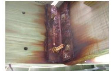
Severely Corroded Connections
