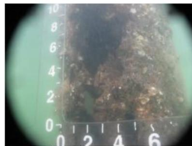
Timber Pile with Severe Marine Borer Damage
