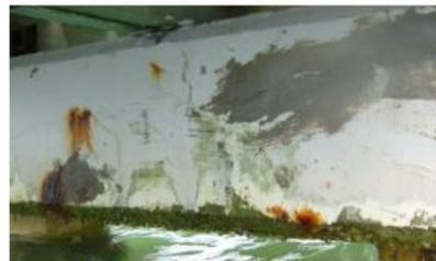
Concrete Pile Cap with Closed Corrosion Spalls
