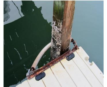
Corroded Connection and Weathered Guide Pile
