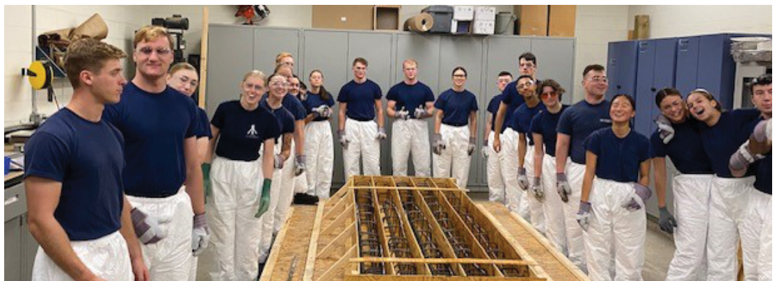
Cadets in the course, 1411 Reinforced Concrete Design, design beams meeting typical failure mechanisms in reinforced concrete. Here, cadets are gathered around the formwork containing rebar, just before placing concrete to produce five beams.
